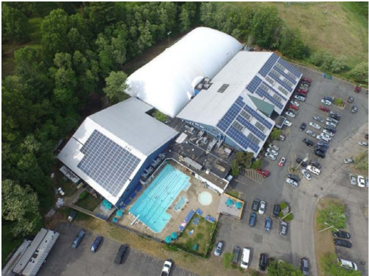
Solect Energy installed solar panels installed on the roofs of the Longfellow Tennis & Health Club in Wayland, MA
