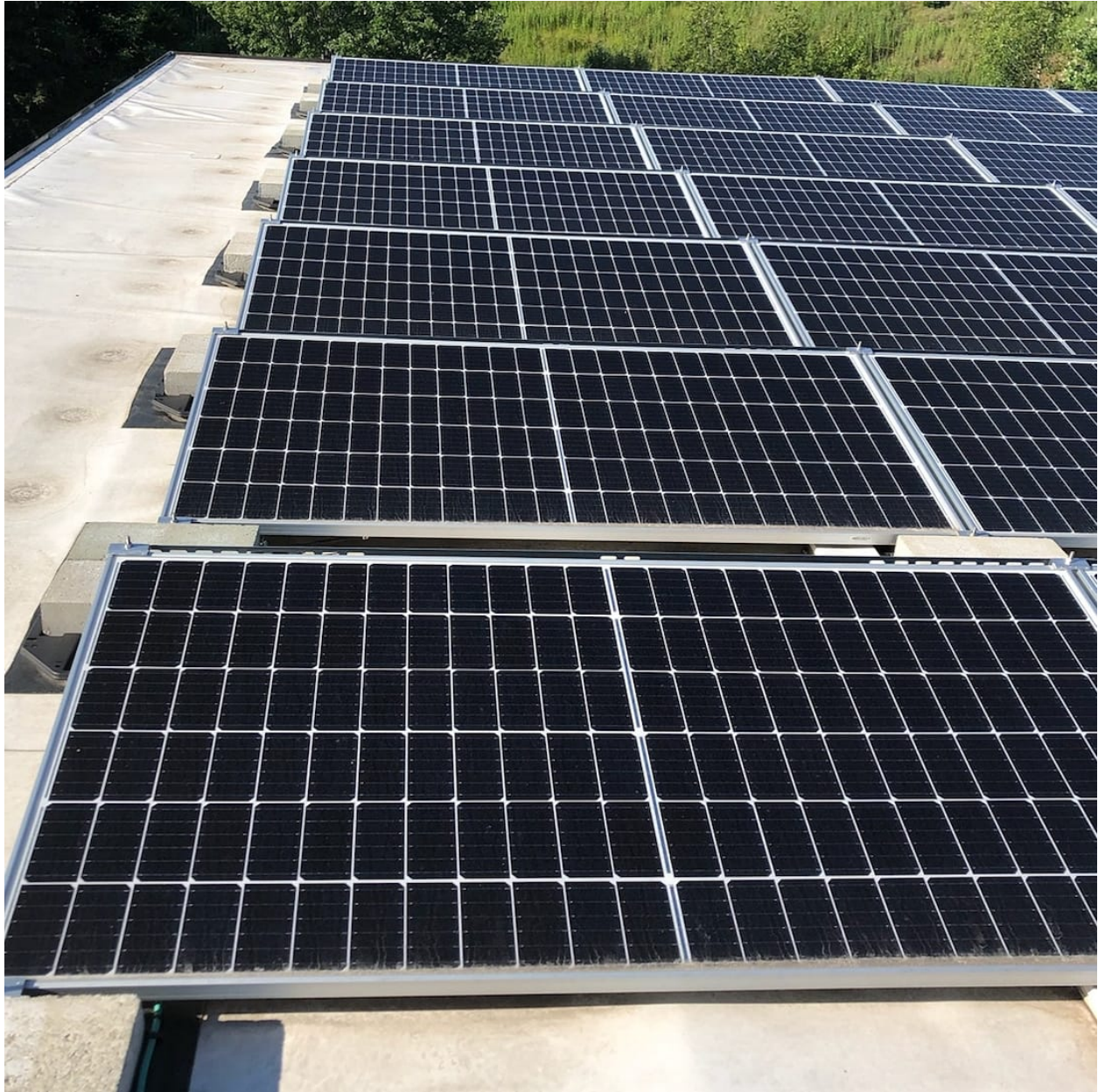
Figure 2. 7th Wave Brewery's 500-kilowatt Solar Array. 7th Wave Brewery. Image of Solar Array. Facebook , 22 Apr. 2021, www.facebook.com/7thwavebrewing/photos/2080382228770745 .
